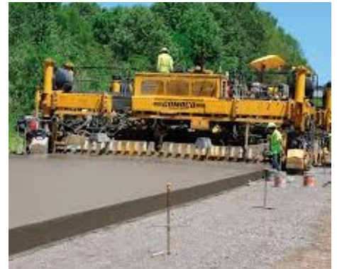
Road will be constructed by slip-form paving equipment.
