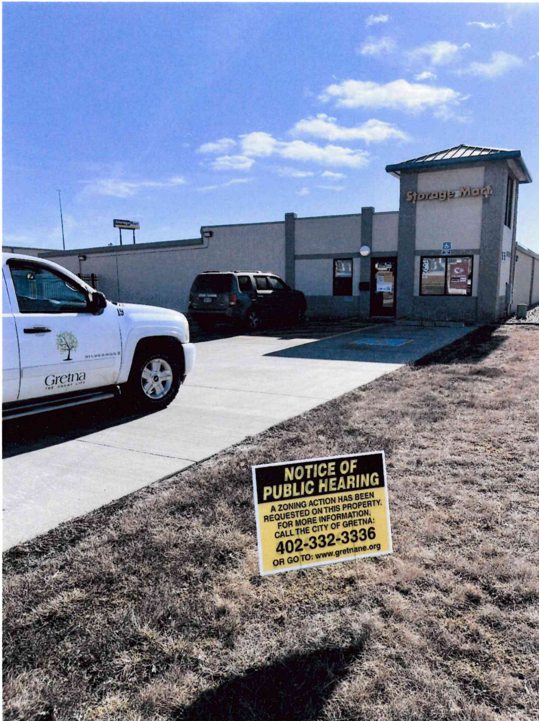
Lot 1, 370 STORAGE (11001 Sapp Brothers Drive) facing East.
