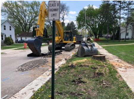
Concrete panel removal
