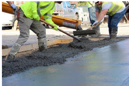
Concrete will be repaved in areas of removal
